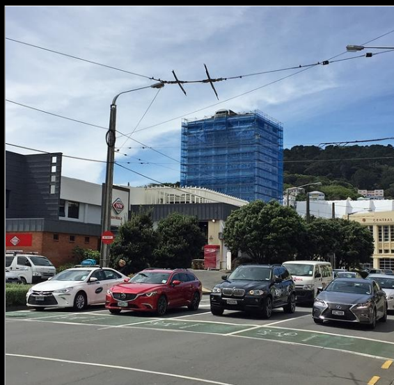
Right: Peter Grove's letter refers to the $11 million cost of removing the overhead. Ten days after the publication of his letter this was the scene in Wakefield Street on 26 October looking towards the intersection with Taranaki Street. An "End of an Era" board remains on the traction pole and a couple of span wires with a 'Slow' sign ahead of where switch 403 once was are all that's left to remind us that trolleybuses ever came this way.
